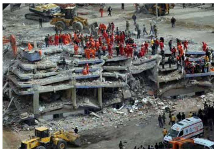
An aerial view taken from a helicopter shows rescue teams trying to salvage people from a collapsed building after a powerful earthquake rocked eastern Turkey, in Ercis district in Van, on 25 October 2011
